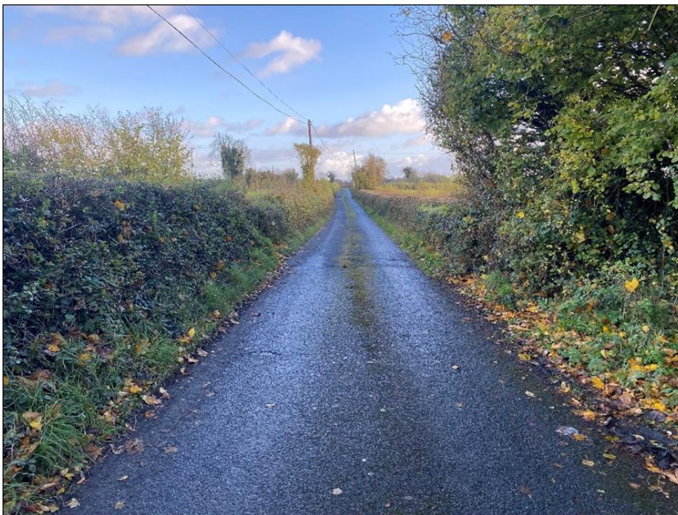
Plate 3-29 Route for grid connection underground cabling on road crossing at Clonmore river bridge located at the south east of the Site.
